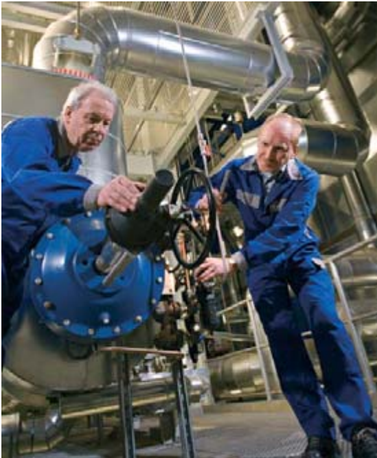
Service Engineers commissioning a desuperheater and steam conditioning valve.
